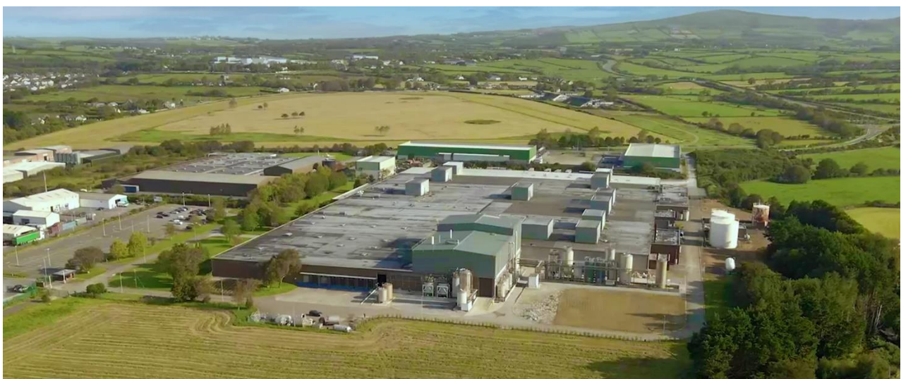
Figure 30. Facilities of BioAtlantis in Kerry, Ireland (Source: https://www.bioatlantis.com/ ).
