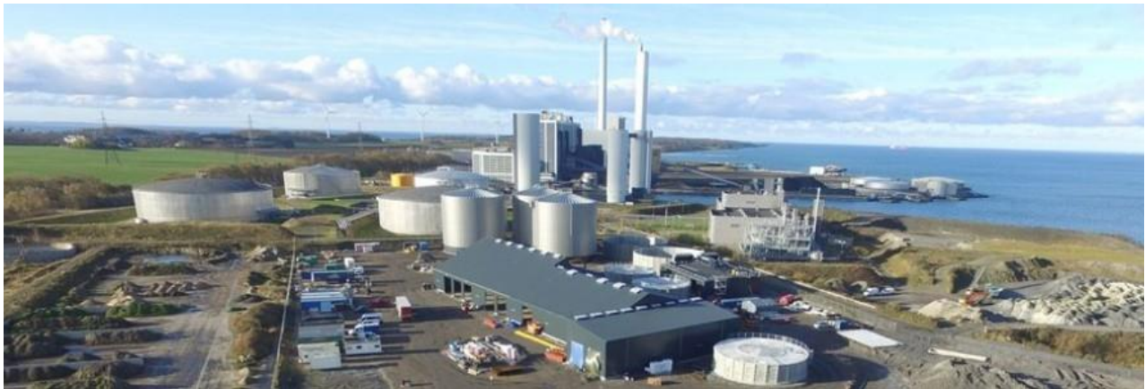
Figure 18. Maabjerg BioEnergy biogas plant based in Holstebro Denmark (source: https://bigadan.com/ ).
