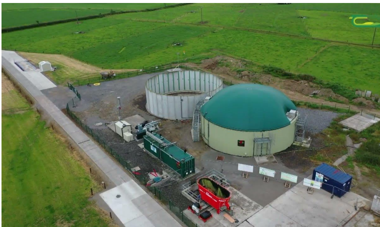
Figure 26. Teagasc Grange Biogas Plant at Grange, Ireland (Source: https://www.teagasc.ie/ ).
